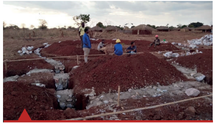
Beginning of the construction of the Guy Reinaud Rural Center for Agroecology.
