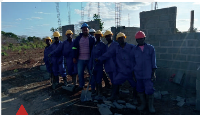
Construction team at the Rural Center.
