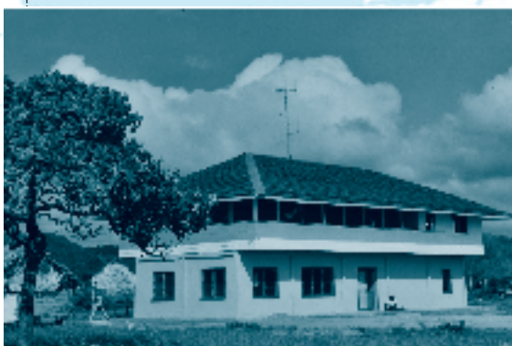
Bina Hill Institute for Research, Training and Development, Region 9, Guyana - main building.
